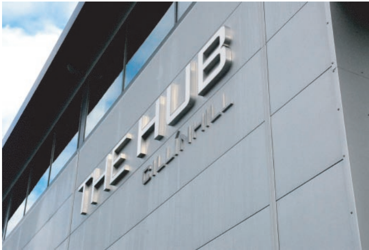
The Hub, Cillín Hill, Kilkenny Stainless Steel Built-up letters with Acrylic internally lit face
